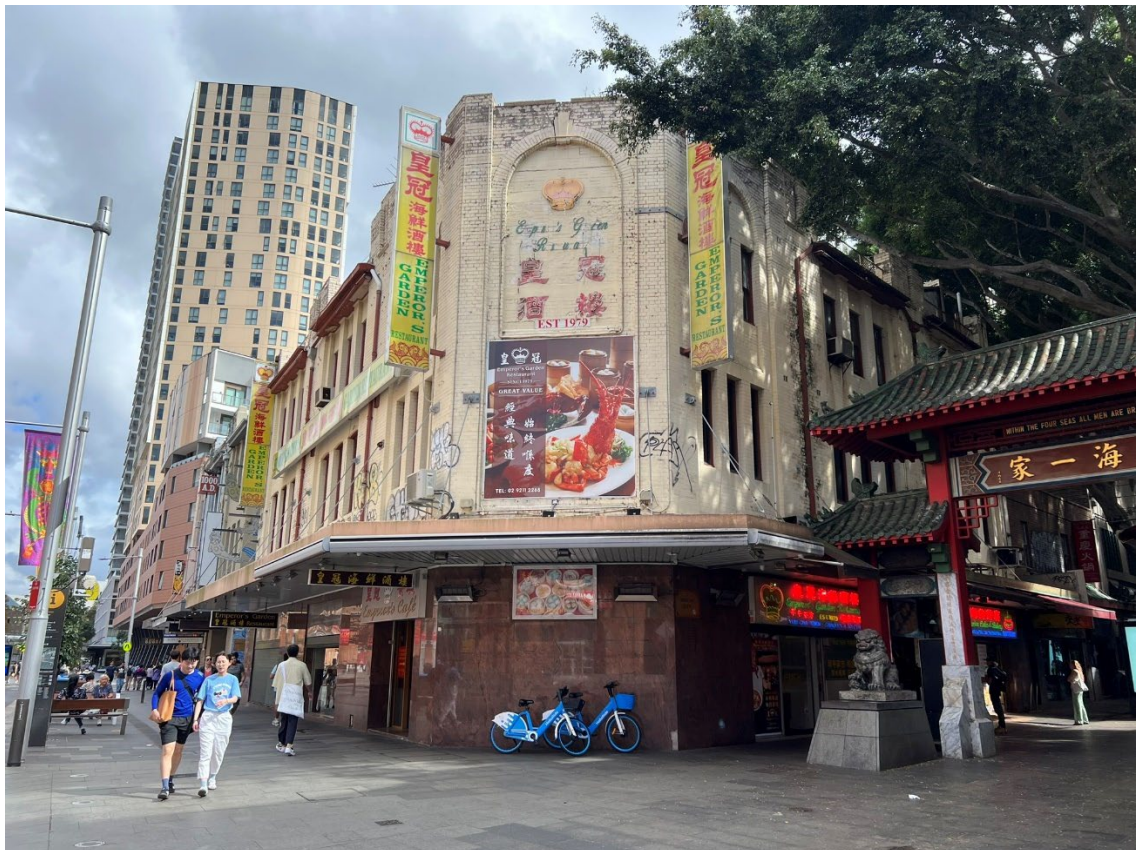
Figure 37 No. 100 Hay Street with its chamfered corner and arches and balustrades to the central and north bay to Dixon Street.
